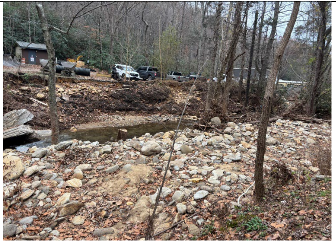
B-2. View across Flat Creek showing emergency stone ballast on west bank. This is part of the project site needing further bank restoration.
