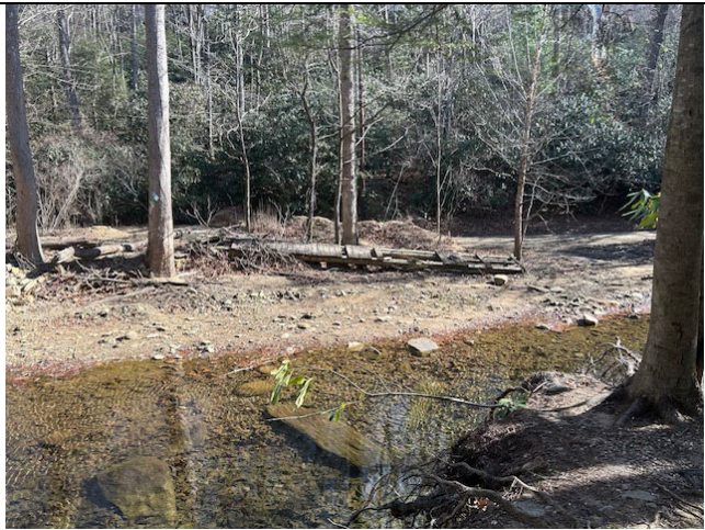
B-3. Broken footbridge resting on eroded creek bank
