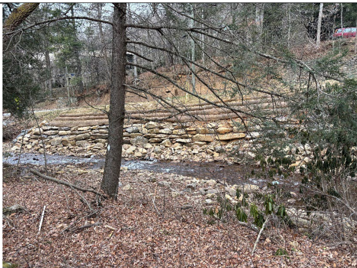
B-5. This is one section of restored creek bank upstream from the project site showing the geolift system repair.
