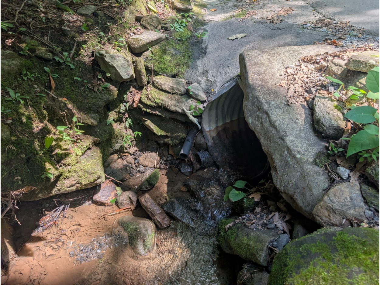
Figure 2. Looking upstream at culvert outlet on east side of Kentucky Rd.
