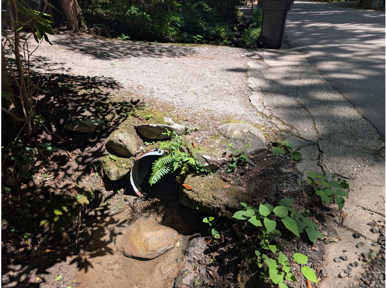
Figure 1. Looking downstream at culvert inlet on east side of Kentucky Road.
