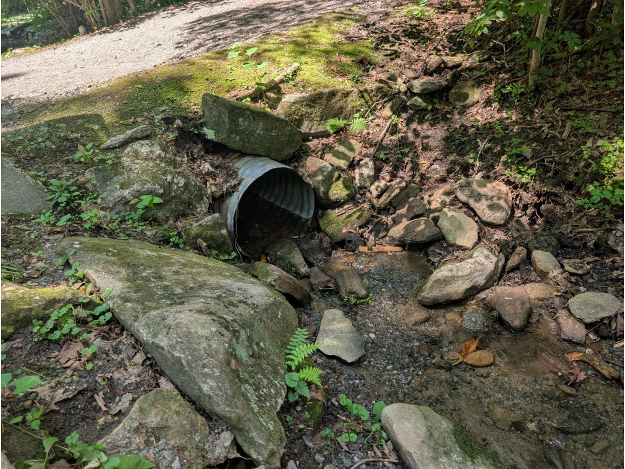
Figure 4. Looking downstream at culvert inlet and southern adjacent property.
