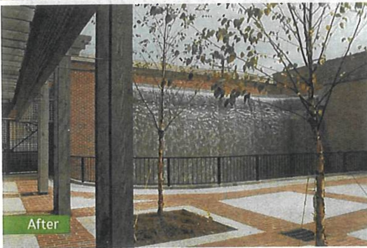
The 45-foot-wide, curved "pocket" waterfall was constructed and pretested before installation.
