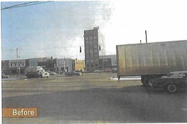
A view of the gauntlet of asphalt, trucks, and trains that pedestrians faced prior to the project.
