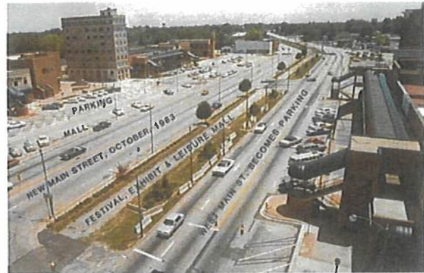
Midway through the project: the N&S Railroad was relocated 3 blocks to the north. Two-level arcades were added to 3 city blocks.
