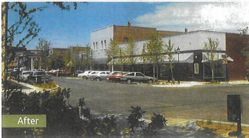
June 1983 — Ugly elements are removed, brick cleaned, windows repaired, new storefronts and awnings install, and perpetually maintained by the owners, according to the ordinance.
