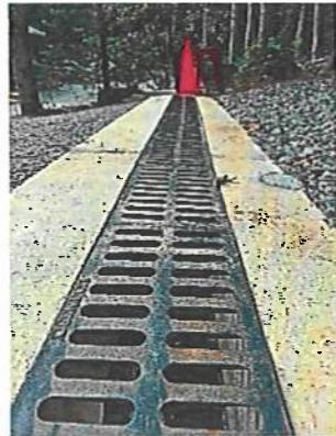
8. Installed twelve tons of railroad ballast stone above the new fifteen-foot catch basin to catch potential gravel erosion from the uphill neighbor's lot.
