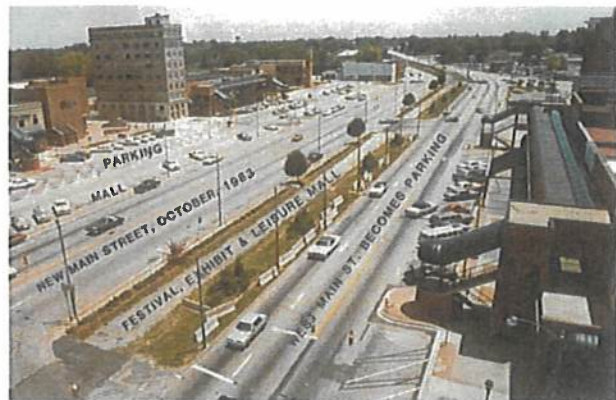
Midway through the project: the N&S Railroad was relocated 3 blocks to the north. Two-level arcades were added to 3 city blocks.
