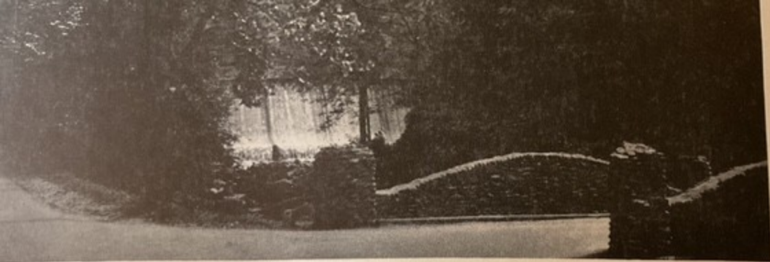
Overflow of Lake Susan. Hard surface road and concrete bridge.
