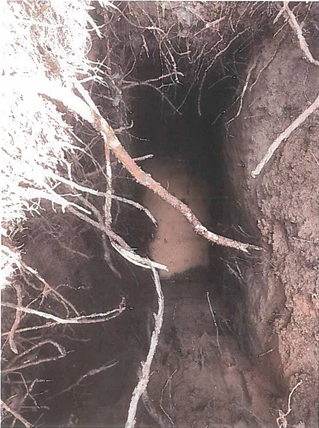
Photo 6 – Test Pit 2 at 8 to 10 feet
